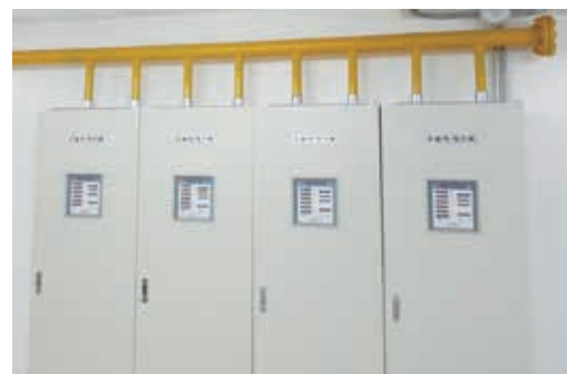
[ Installation of modular system ]
