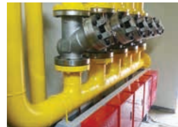
[ installation of selection valve ]
