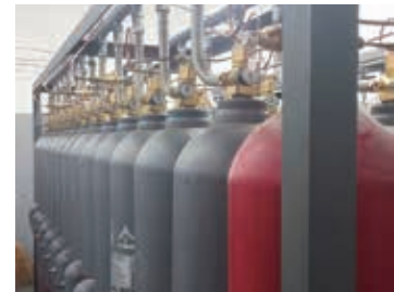
[ completed collecting pipe of cylinder ]
